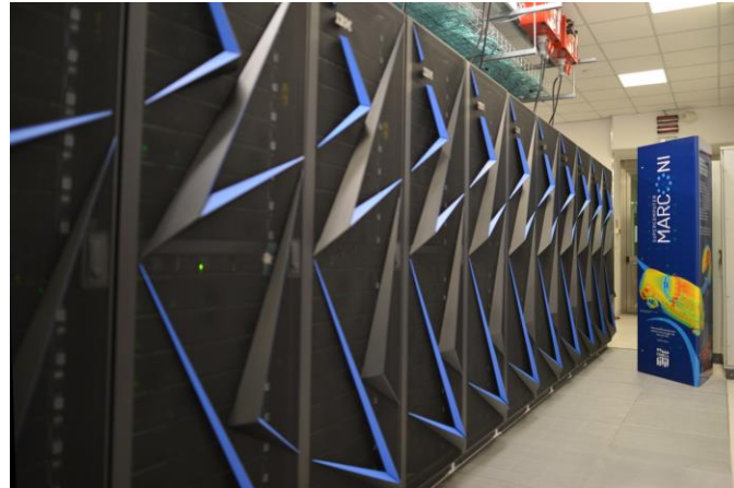
#9* Marconi100 – IBM Power9 + Nvidia V100
